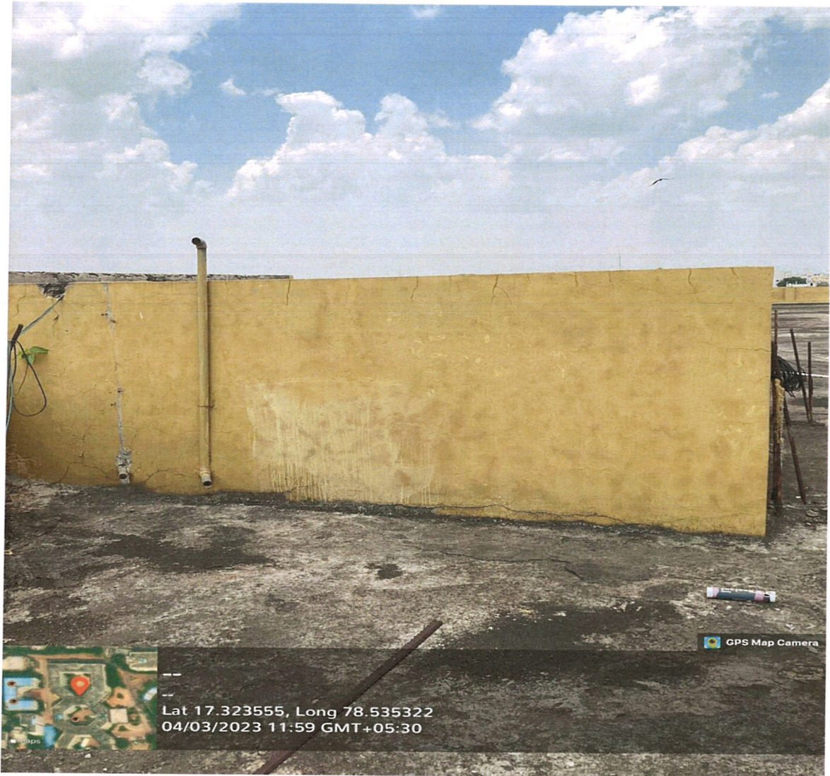
Water Tank for Distributing Water in the campus
