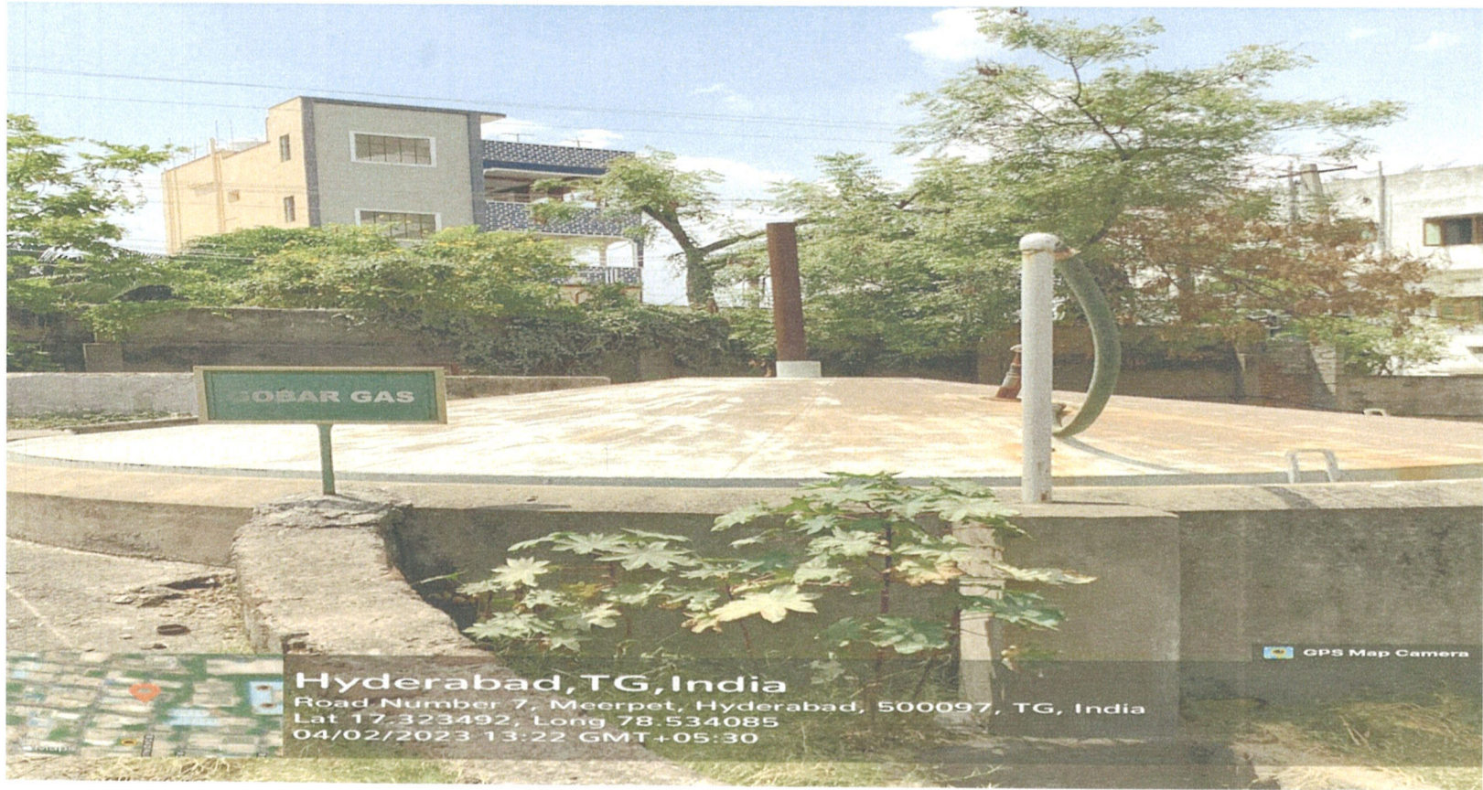
Biogas Plant Unit
