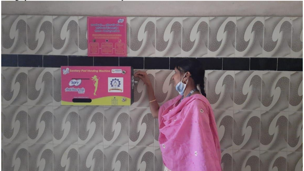
Sanitary Wending Mission installed in College Premises
