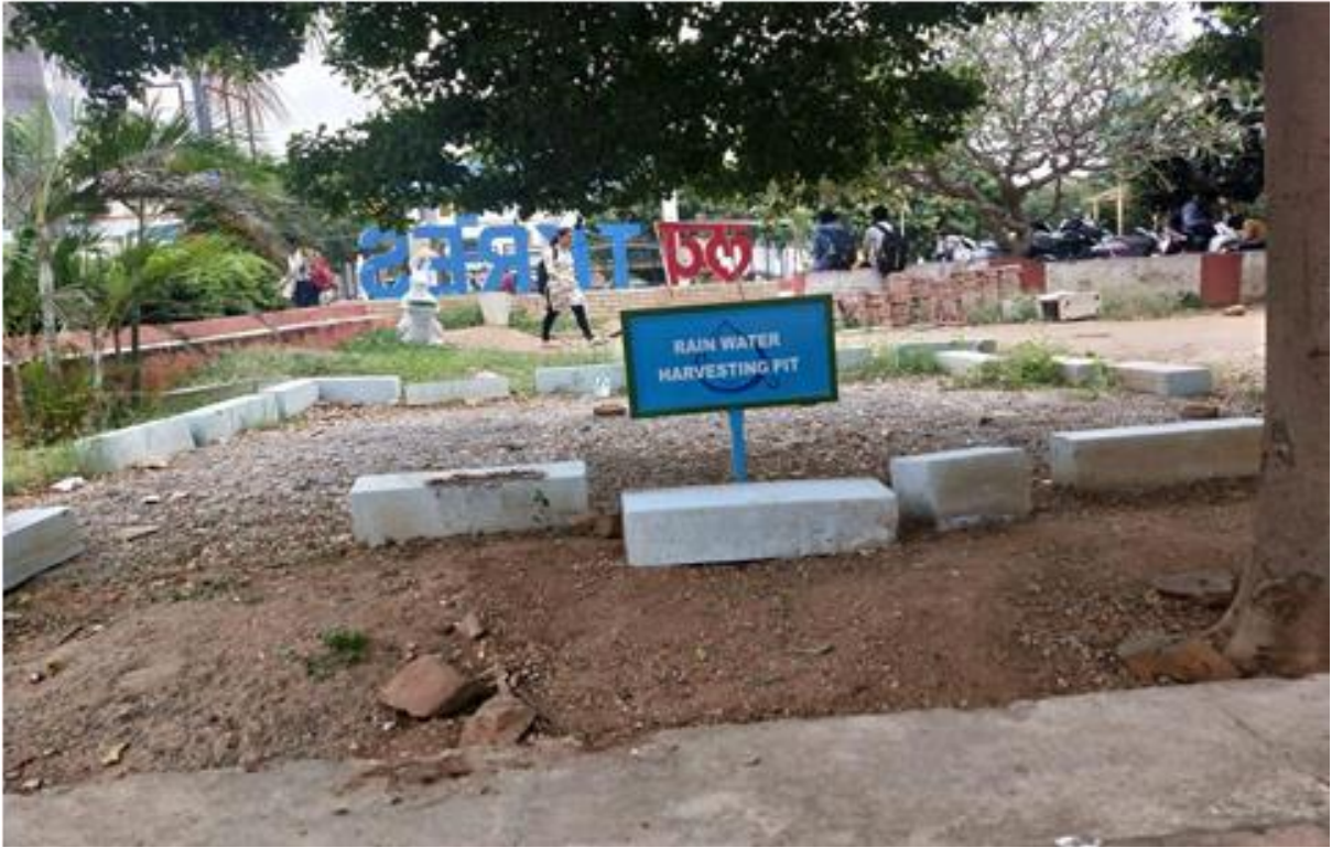
Harvesting Pit-4 in TKRCET
