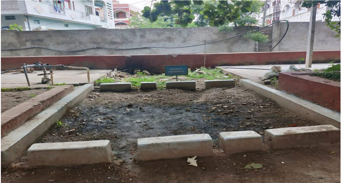
Harvesting Pit-6 in TKRCET
