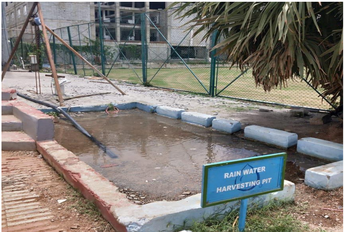
Harvesting Pit-3 in TKRCET
