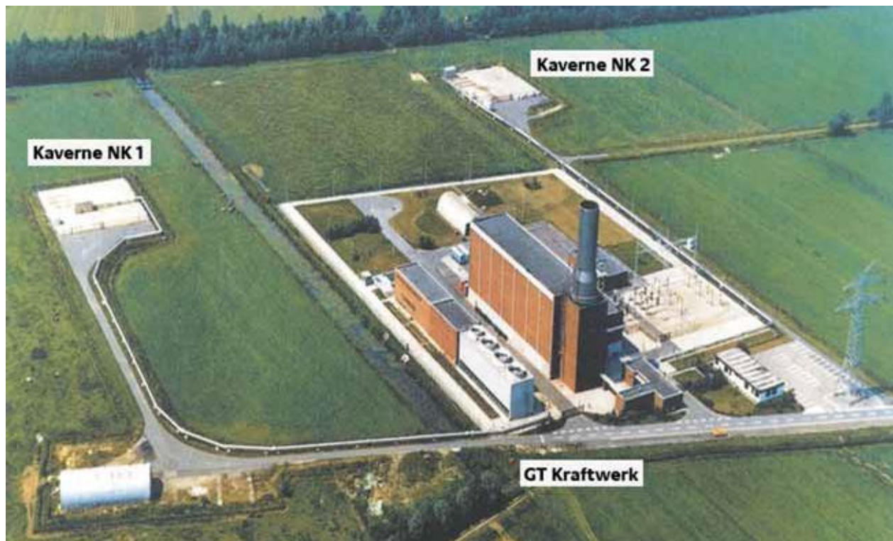
Figure 3-2 | CAES plant in Huntorf ( Vattenfall, IEC MSB/EES Workshop 2011 )
